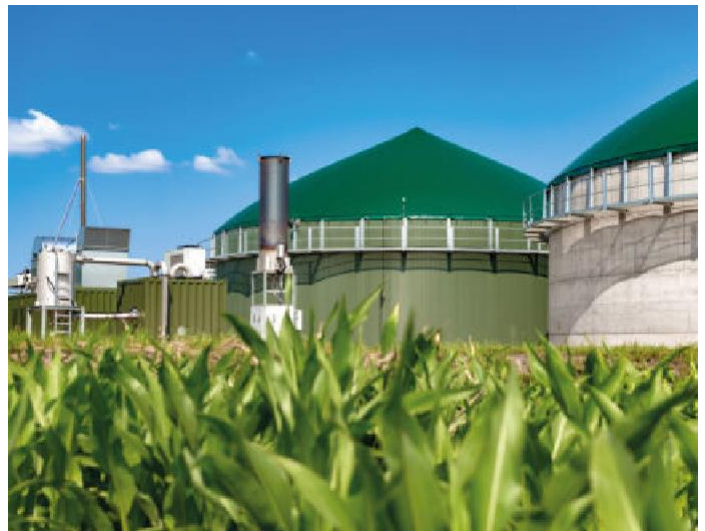
Agricultural biogas plant
